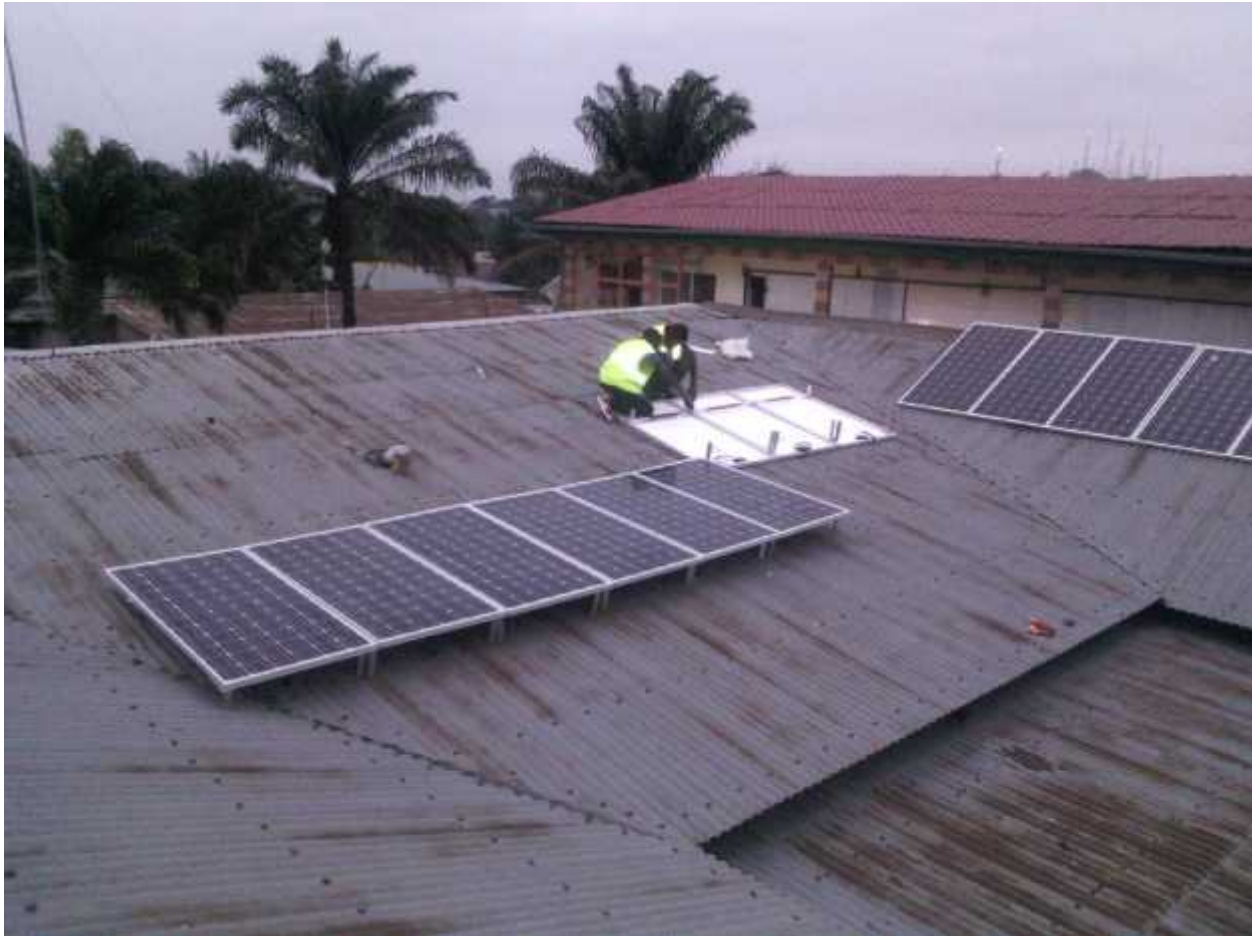
SMIN Power Group technicians installing a solar system in D.R.Congo.
