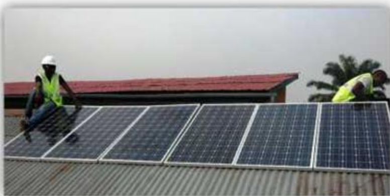
Fig.1: SMIN Power Group technicians installing rooftop solar system.
